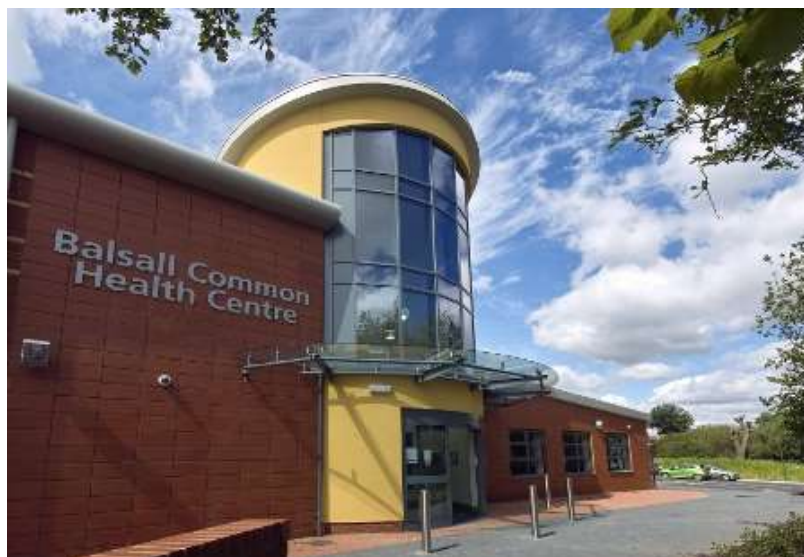
Balsall Common Health Centre
