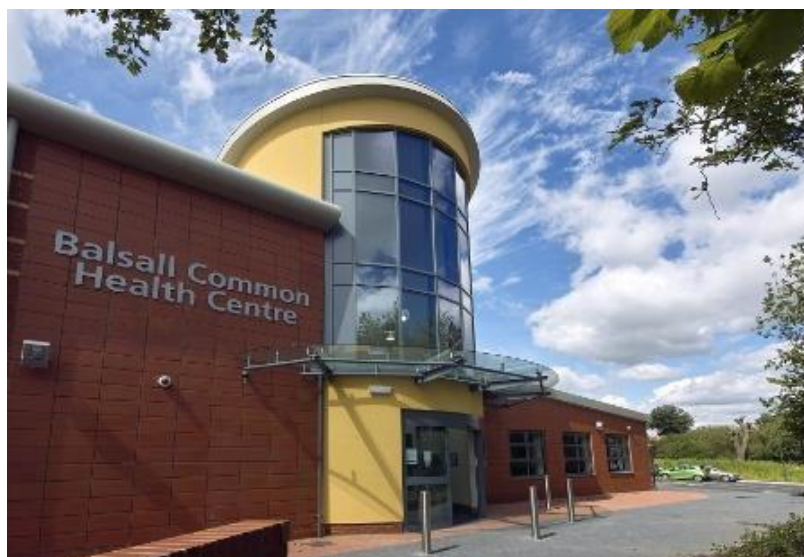
Balsall Common Health Centre
